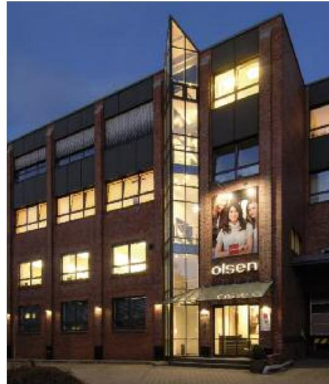
The addition of two storeys onto the building in the 1980s resulted in the converted storey – in those days the topmost production floor – being fitted with the additional supports and joists necessary for structural stability. The difficult part for the architects was to transform the dominant static structure into an attractive, clear and open space concept.
