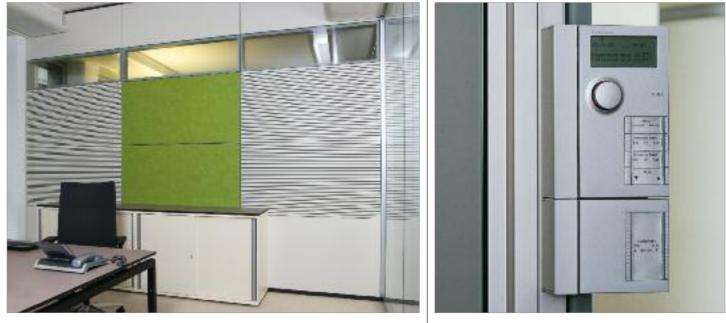
elements combining both design and function. In addition to attractive appearance, flexibility and transparency, they also cater in the Spreepalais for high standards of sound insulation, fire safety and sound absorption. Furthermore, additional functions such as LED lights and smoke extraction flaps are integrated into the partition wall systems.
